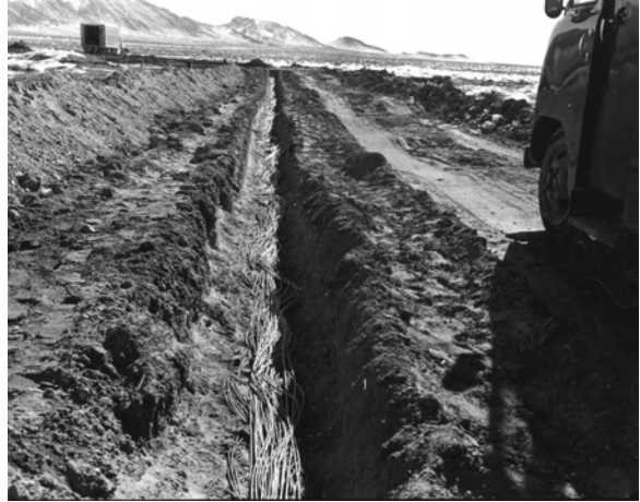
12-1 - Project 1.7.1 26Jan55 Cables laying in trench
